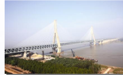
Tianxingzhou Yangtze River Bridge
